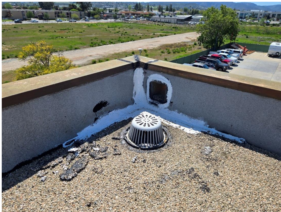
Roof Drain and Scupper Location on Southwest Corner of Roof
