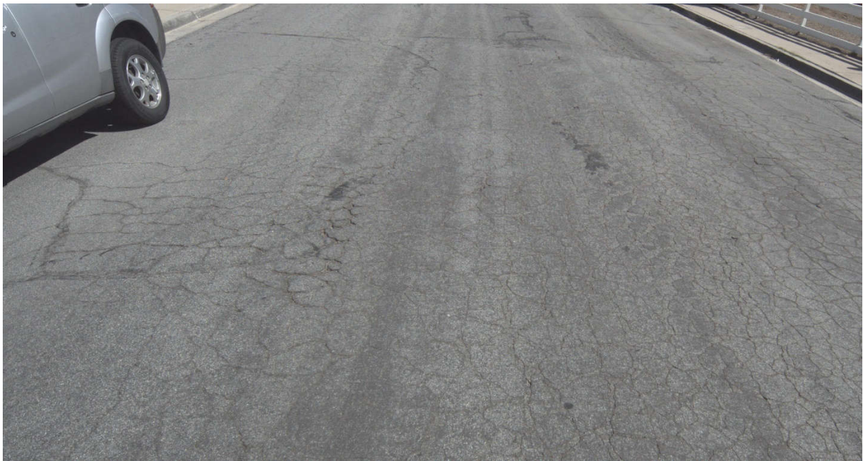
Figure 2. Lutheran Way, Street Number 4050, Block Number 50
