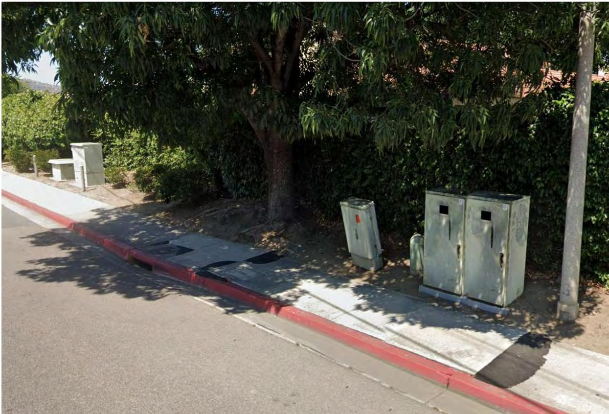
*Example of the temporary ramping repairs caused by tree root intrusion. The tree was evaluated and could not be preserved without potential future damage.*
