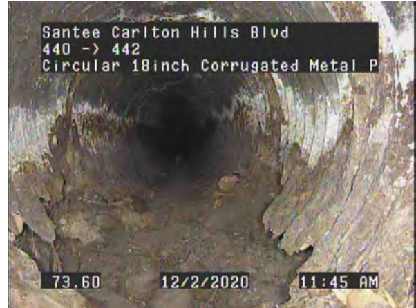
73.60ft Hole Soil Visible from 4 o'clock to 8 o'clock
