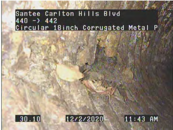
30.10ft Hole Soil Visible from 7 o'clock to 8 o'clock
