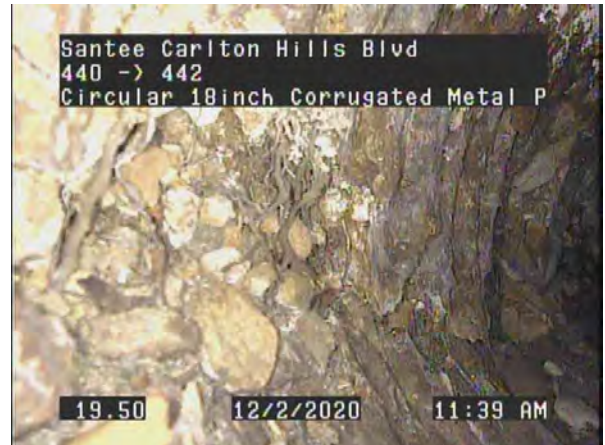
19.50ft Hole Soil Visible from 7 o'clock to 9 o'clock, Start
