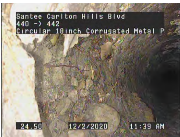
24.50ft Hole Soil Visible from 7 o'clock to 9 o'clock, Finish
