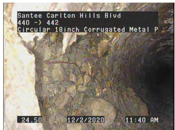
24.50ft Hole Soil Visible from 6 o'clock to 8 o'clock
